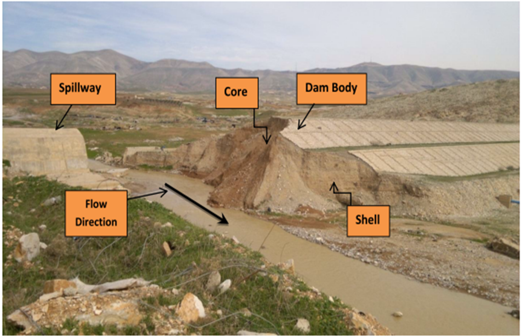
Figure 2: Photo of Chaq- Chaq dam after failure.
